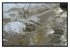
Breaking ice dams is difficult. Sometimes all that can be done is to plow or scrape the snow off the top of the ice and let the sun hit the ice in hopes that it will melt and allow water to run off before spring rains wash the road out. The above situation called for hand chipping the ice to allow water to get to the road ditch and culvert.
