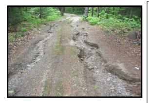
These washouts are the result of lack of maintenance in time to smooth out the wheel tracks caused by everyone driving in the same location (double ruts). Heavy rains followed the tracks even though this is only a gradual slope.
