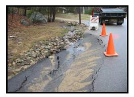
These two photos show water damages to the edges of paved roads due to poor ditch stabilization at the side.
