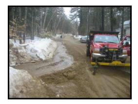
The emergency repair required redirecting the stream back to the ditch to prevent further road damage and allow traffic to pass.
