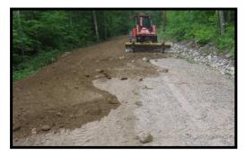
Cutting too deep into the surface of many roads can dig up rocks from the base that might be too big to reincorporate in the crown of the road and would better off left in place rather than lost to the side of the road during cleanup
