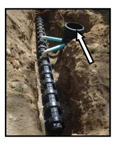
Photo at left shows several "Infiltrator" plastic leaching chambers typically used in septic systems installed in a trench that was dug deep enough to place it in the most porous soil layer available above water table. Stormwater is picked up by the vertical 18" culvert (arrow) and flows into the Infiltrators through the two 4" pipes.
