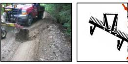
With a rear mounted rake or blade you can usually raise it then back over the berm, drop the attachment and pull the berm back into the road where material can be reclaimed.
