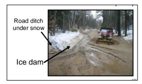
This development road washed out because water could not reach the ditch at left and required some emergency repair.
