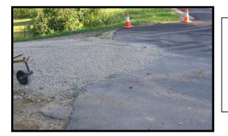
Though having some gravel cover the asphalt in a V or "hip roof" configuration may look like a mistake, it is an effective technique to reduce potholes at the gravel to pavement transition.
