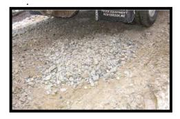
Small pockets of mud or mudholes can usually be repaired with the addition of crushed stone in the same manner as deep muddy roads (11.1.2). If the source of the problem is an active spring, however, it is preferable to install a subsurface drain to remove the water from the roadbed >>see: 3.2 Subsurface Drains<<
