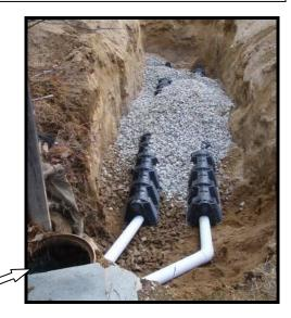
Lower two photos show a low cost addition to an existing catch basin constructed in very porous river gravel. The trench was excavated, the rocks raked out of the excavated material and placed back in the trench with two distribution pipes run out of the catch basin on top of the rocks which are then covered with filter fabric and backfilled.
