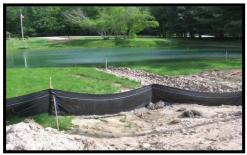
Road construction site bordered by properly installed silt fence
