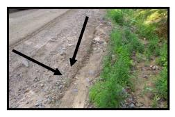
Permanent grader berm left during years of poor grading practices. Note the ditch at right, but water is forced to traveling IN the road. (arrows)
