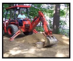
Constructing the Rolling Dip-digging a low spot across the road with bucket or, in this case, the backhoe blade
