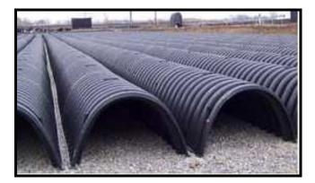
This is an example of a large scale storm water storage and infiltration system being installed under a municipal or a large mall parking lot to return stormwater to the ground
