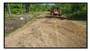
For this driveway reconstruction, shoulders have been pulled in with a tractor to form a substantial "lift" in the middle of the road and grading has begun
