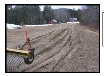
Soft road surfaces can be reinforced with the addition of clean crushed stone, not crushed gravel (see text 4.1). (see photos next page)
