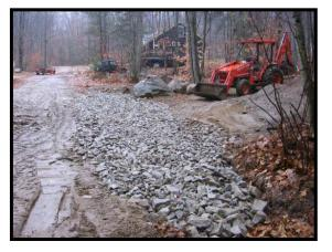
Another dip at the side of a development road across a private driveway with a substantial springtime flow across it, before surface gravel was added. Note the largest stone is 6" with 3" and 1.5" stone filling the voids. <sup>3</sup>/<sub>4</sub>" gravel forms the final surface, filling remaining voids, so that the stone disappears and the surface is smooth and firm to walk and drive on, but running water cannot erode the stone.
