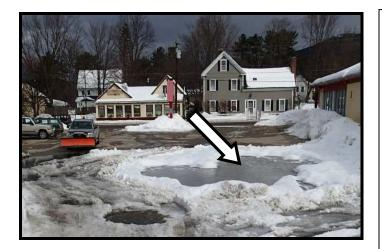
The catch basin in the middle of this large parking lot has been plugged for years making the lot extremely difficult to maintain in winter as well as a challenge for those who have to drive through it when there is over a foot of standing water and ice chunks. Arrow points to the submerged catch basin in late March 2014. It looks like the snowplow contractor gave up trying to clear around the basin after the last snowstorm since it is impossible to plow!!
