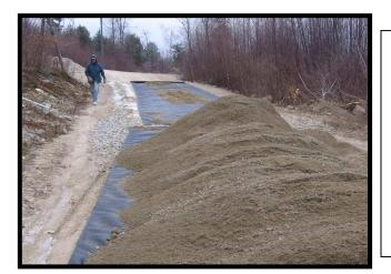
Geotextiles keep the gravel on top from being pushed down into the soil underneath, compensating for a poor road base
