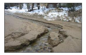
Although only certain roads provide direct access to ponds, lakes, and streams, the runoff from *all* roads eventually finds its way to surface water. Unstable roads become channels through which sediments and nutrients reach sensitive lakes and ponds, causing significant adverse effect on water quality.
