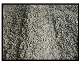
Here <sup>3</sup>/<sub>4</sub>" stone is being added and worked in with the grader/rake to form a strong surface that resists rutting
