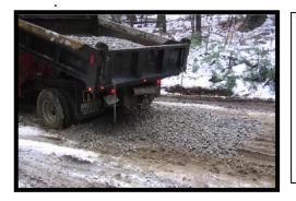
If a road turns to impassible mud in the spring, the only practical way to return it to service immediately is to add crushed stone (not gravel) to strengthen it. Use larger ( $1\frac{1}{2}$ " stone) until road firms up. It's generally cheaper and stronger than  $\frac{3}{4}$  stone. Stone is worked into the mud until the road is able to support passing loads. Though expensive, this scheme is very effective for emergency repairs.
