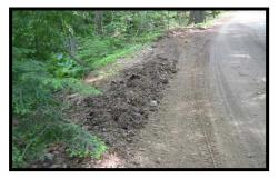
Grader berm left during grading
