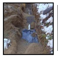
Installation of an underdrain on the uphill side of a private driveway to remove groundwater
