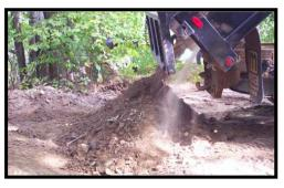
Adding "ditch mix" that consists of several sizes of crushed stone from several inches down to small stone and some fines to hold it together. "Tailings" from a gravel producer can work very well for this purpose. Otherwise, mix several sizes of stone together, sometimes as large as 6" depending on the application. This particular crossing was lined with tailings.
